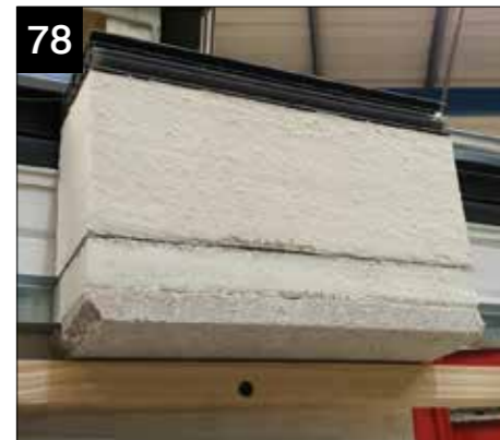
78 Above the walled areas access is restricted for fixing chosen internal boards to the ceiling. It may be required to use the battening to construct a small frame or to fix batten into the firrings to act as support for the boarding. The Garden Room installation is complete and internal boarding and finishing can commence.
