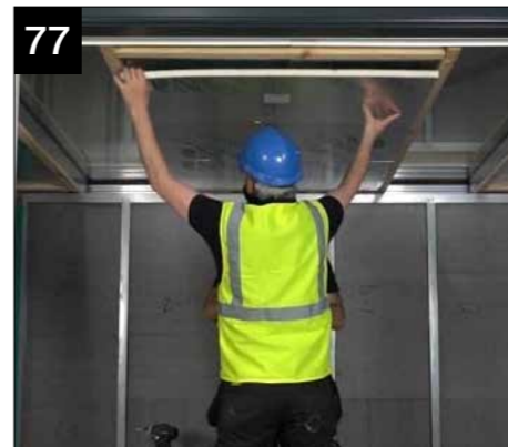
77 Next fit the 25mm insulation board. These boards must be laid at right angles to the glazing bars and run across the bars. Fix in position using LVIK025 fixing kit. Seal the joints using the foil tape (LVFT045).
