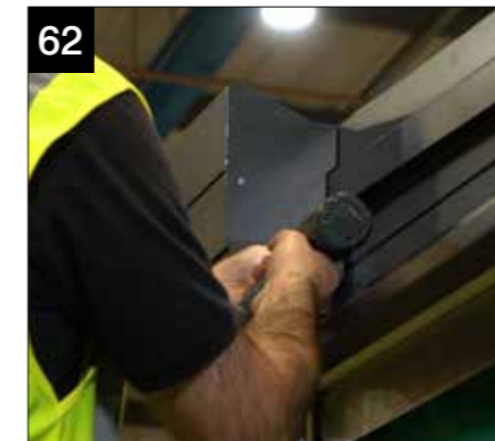
Fit cornice end caps on both sides using the provided screws 8PSR42-25BLK.
