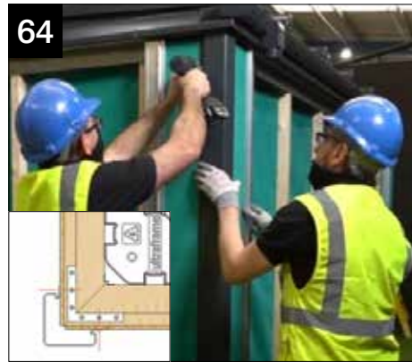
64 Position corner against column ensuring it is a good tight fit against the underside cornice/cill. Screw fix through holes into column using the 4.8 x 25mm pozi pan screws supplied (EFSA021).
