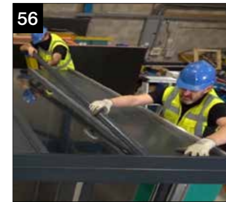
Position bar top cap. Using the heel of your hand, push down on the top cap to engage the clips, working from cornice to eaves. Ensure the rubber gaskets are fully compressed for a watertight seal and that the top caps are up against the cornice section. NOTE: on longer bars it may be necessary to use a soft mallet and timber block.
