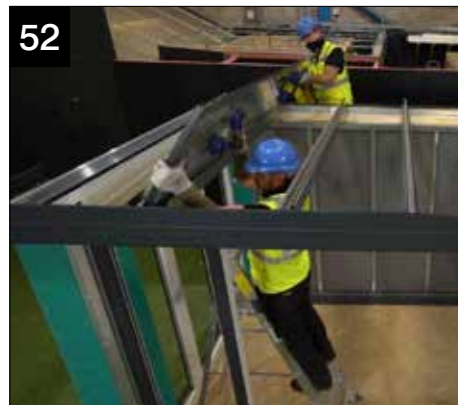
Position the panels and glazing onto the roofing bars and centralise. Pushing up as high as possible against the upper cornice. If necessary pack it out on each side.
