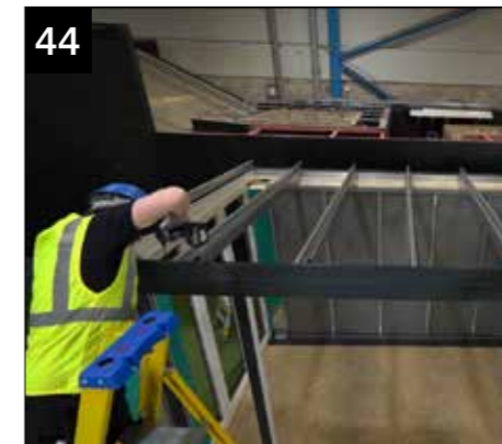
Offer up the cornice upper sections fixing inline with the glazing bars centres using CHA007. The upper sections do not require the corner cleat. The corner end caps perform this function.
