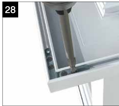
Secure these cleats in place using (CHA007) fixings provided.
