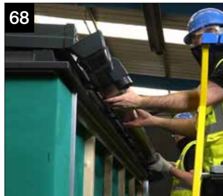
68 Decide on the location of the outlet. Assemble the gutter, brackets, stop end and stop end outlet and lift into position on the external fascia. Push down to locate the lower leg of the bracket. Assemble the rain water pipe, attach to the gutter and screw the down pipe bracket to the frame.
