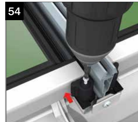
Pushing the glazing/panel up against the upper cornice. Using the fixings provided, screw down the glazing stop into the bar as shown. Now fully peel away protective film from glazing support at eaves and press glazing down firmly.
