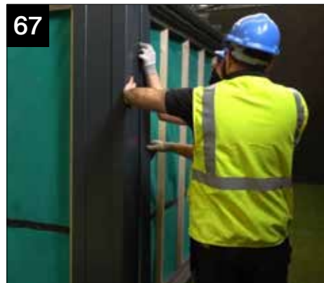
67 Clip on cladding as shown by locating inside clip first and rocking over the external clip. This motion may be more difficult where the cill terminates into the side of the column, it may require a gentle tap to engage the clip. External claddings of choice can now be fitted to the walls.
