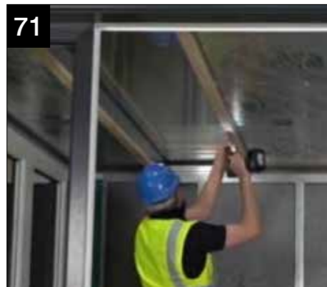
71 Down each side of glazed area and perpendicular to the glazing bars at the top and bottom end of the solid roof section, attach 25 mm x 40mm batten, ensure it sits 6mm outboard of bolster.
