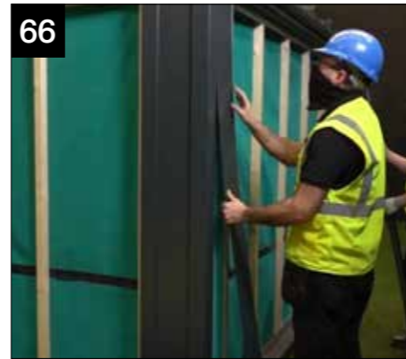
66 Fit powder coated infill panel into one side of the corner cladding and rock back into the cladding clip. Pressing into sealant.
