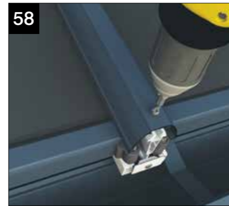
Drill a 6mm hole through the aluminium top cap. Use the fixing provided (CRN010) to attach the top cap to the glazing bar.
