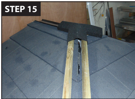
Use the three way cap to set the top, then mark each side of the battens
