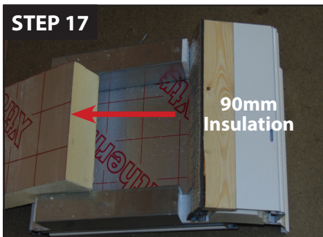
Install the 90mm insulation inbetween the bars inside.
