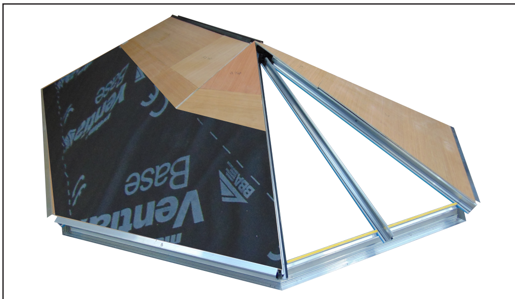
Cover the plywood with a breathable membrane
