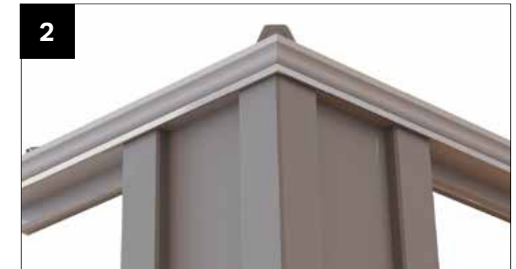
2 Super-insulated columns with Cill
