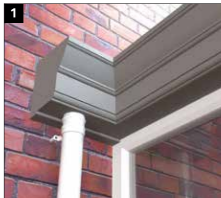
1 Return Cornice and guttering along house wall.
