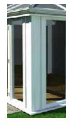
2. A full height structural super insulated columnthat is fully fixed at the base. Detailed on p16 in Super Insulated Column System Overview.
