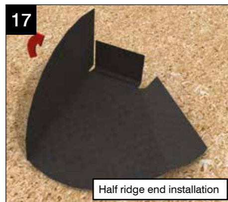
17 The half ridge end flashing detail should be folded as shown and fitted in a similar manner to that of the full ridge end.
