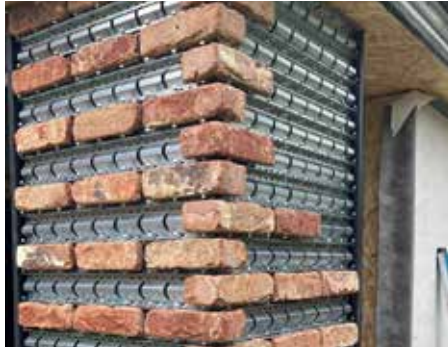
Brick Slips rail application
