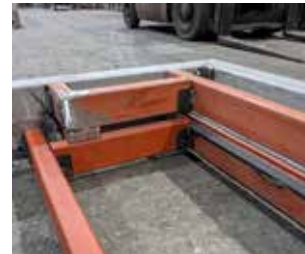
Inner edge beam return to door pocket
