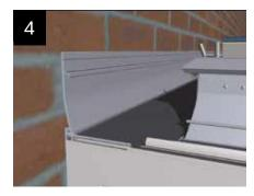
If required, place eaves beam section – with under gutter trim attached onto the side frames. Seal the joint between the eaves beam and box gutter.
